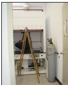
Figure 20: Taiwanese men replacing the hood that was blown up
