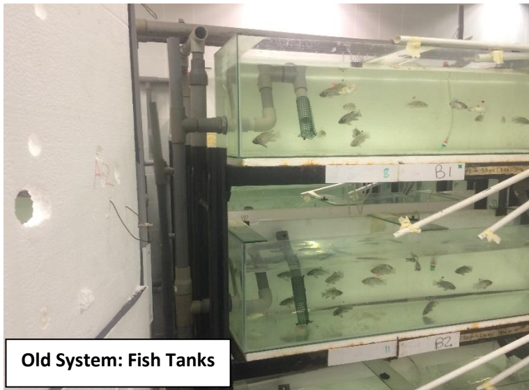
Original Design: Notice the water drains from the fish tanks to the biofilters, then to mechanical filtration
